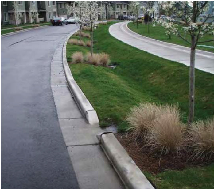
Bioswale | Philadelphia Water Department Stormwater Manual
