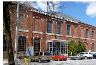
C.H. Evans Pump Station Brewery
