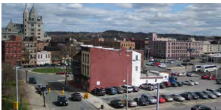
Convention Center site
