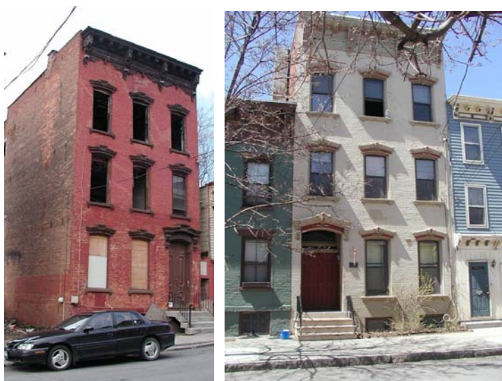
Three story residences: before and after rehabilitation.
