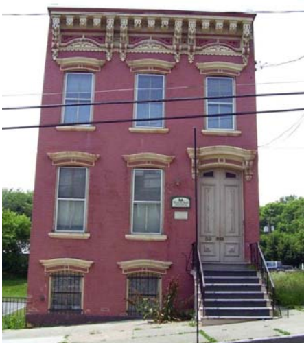
The previous Weed N Seed headquarters on Elizabeth St. at Alexander St.
