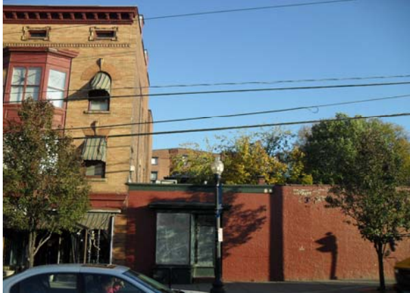
View looking south-east at 423-25 Madison Ave. across Lark Street
