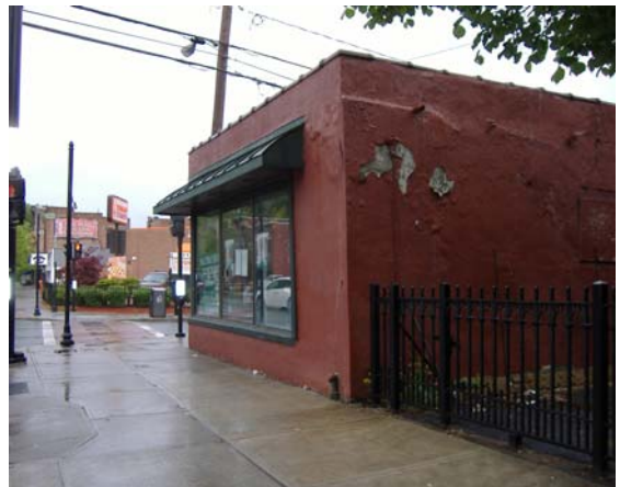
View looking north at 423-25 Madison Ave. from Madison Avenue sidewalk
