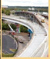
Capitalize Albany Corporation completed its 2018 feasibility study and the Skyway's preliminary-design which readied the project to move forward with construction-ready drawings converting the I-787 northbound exit ramp from Quay Street to Clinton Avenue—into the Region's first and only highline park.
