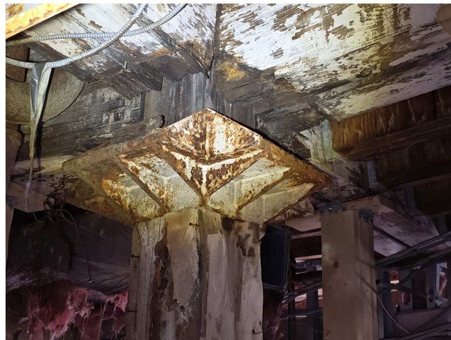
P1 TYPICAL 4WAY COLUMN CAP SCALE: 1" = 1'-0"
